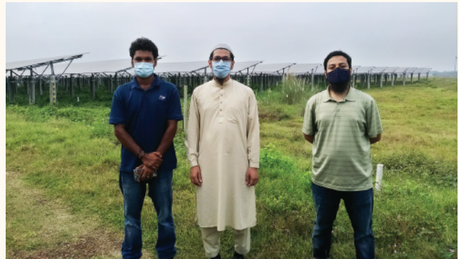
Site Visit at 50 MW Solar Power Plant, Sutiakhali, Mymensingh
