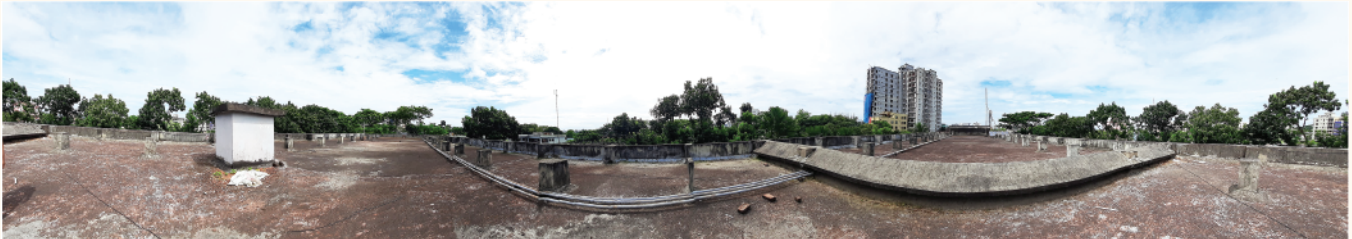
Inspection of the Rooftop of Feni DC Office
